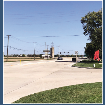
US 34 Widening and Reconstruction
