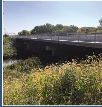
IL 83/US 6 Bridge Replacement over the Little Calumet River
