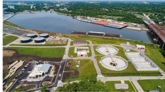
Joliet’s Collaborative Approach to CSOs Mitigates Impacts During Wet-Weather City of Joliet, IL
