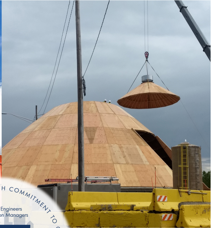
6 Salt Domes & Maintenance Facility Improvements 2020 ACEC Merit Award
