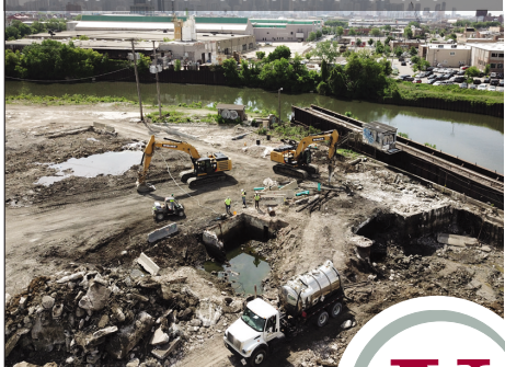
Lincoln Yards North Site Remediation
