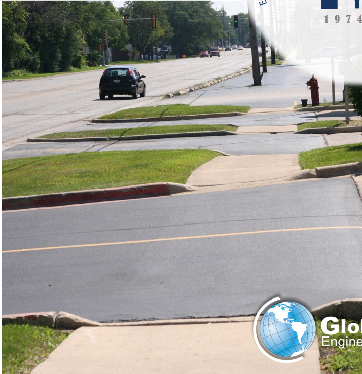
55th St., Safety & Operations Improvement Study 2020 ACEC Merit Award
